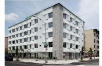
Knickerbocker Commons, the first mid-sized apartment building designed to Passive House standards in the United States
