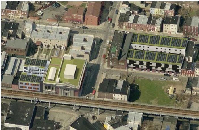
BANK FLATS 2016: 31 units and retail
