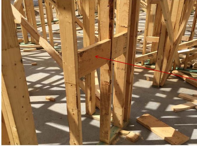
Lumber scrap used as blocking
