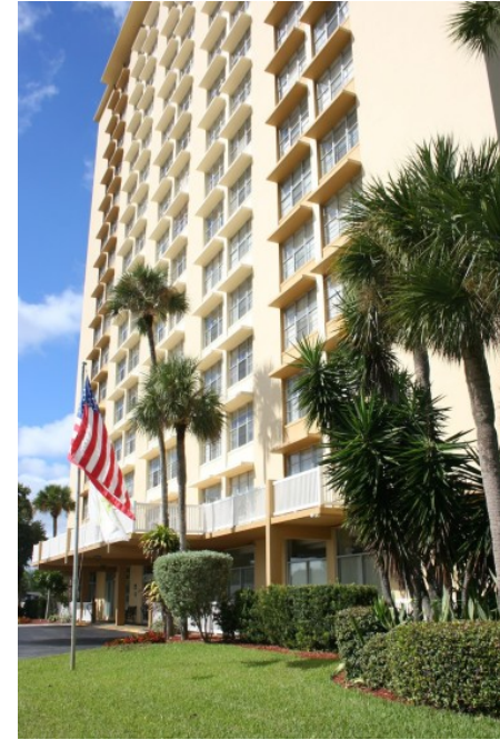
Trinity Towers (192 Units) Melbourne, FL Acq. / Rehab. LIHTC
